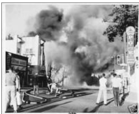
Fire viewed from 4th Street Source: GenDisasters.com
