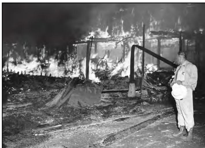
Final destruction Source: MHM
