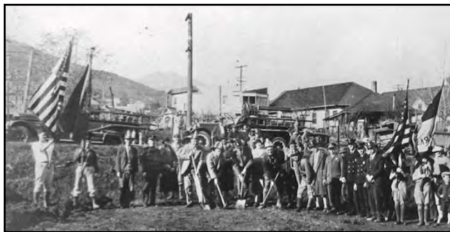
Ground breaking for new firehouse in 1930 Source: MarinFireHistory.org
