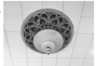
Mechanics Bank ceiling
